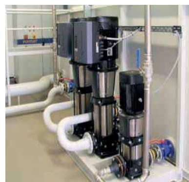
Thanks to flexible modular units such as frequency-controlled machine pumps, tanks and cooling components, the ZFA-system can adapt to changing system requirements
